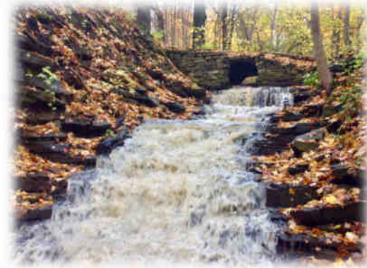
Above: Just west of 30 Rd, by Grimsby, October 27 th , after a heavy rain. Photos: George Prins.
